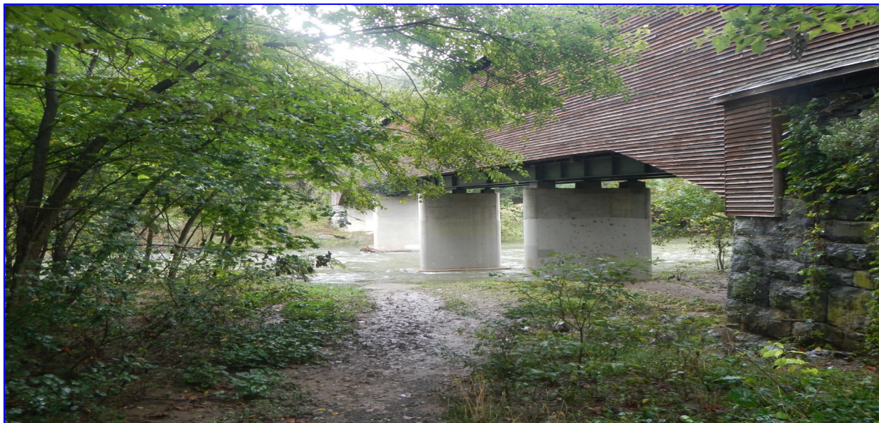
Figure 9: The North Fork Shenandoah River at Meems Bottom Covered Bridge ( FSMB )
